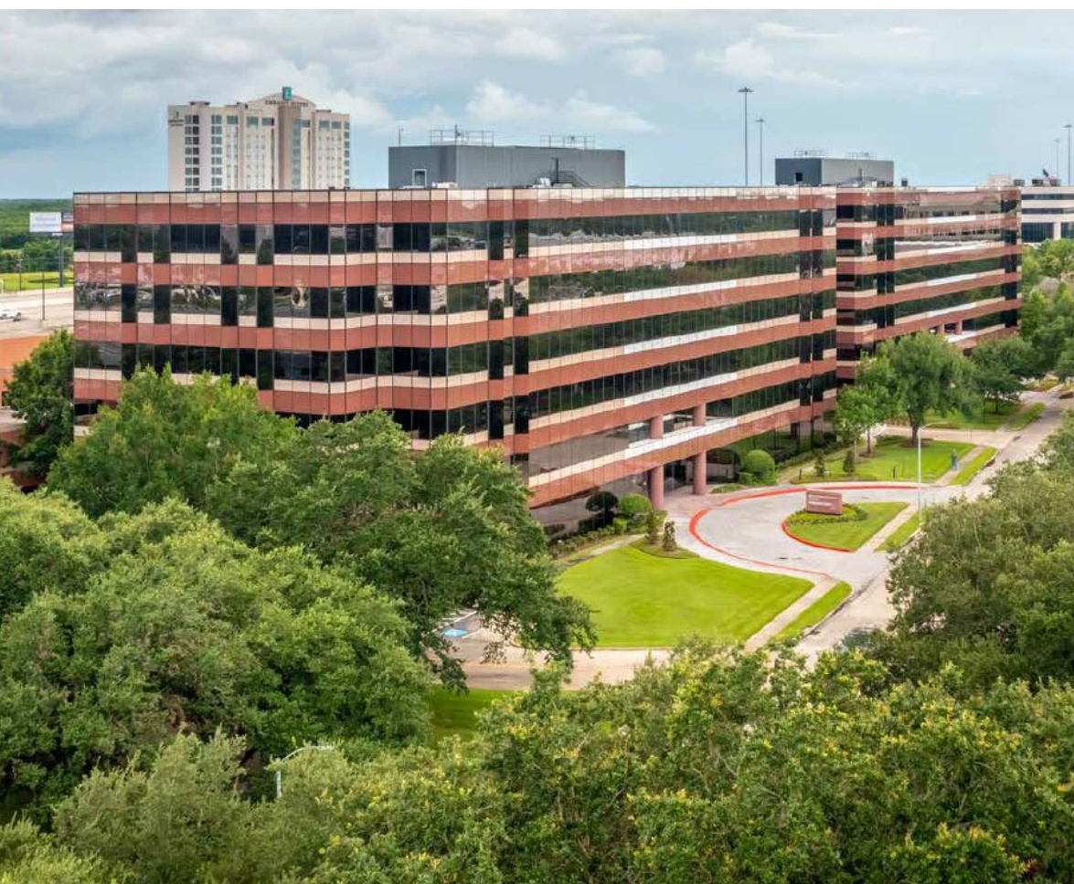
Park Ten Phase II, Houston, TX ENERGY STAR Labeled
